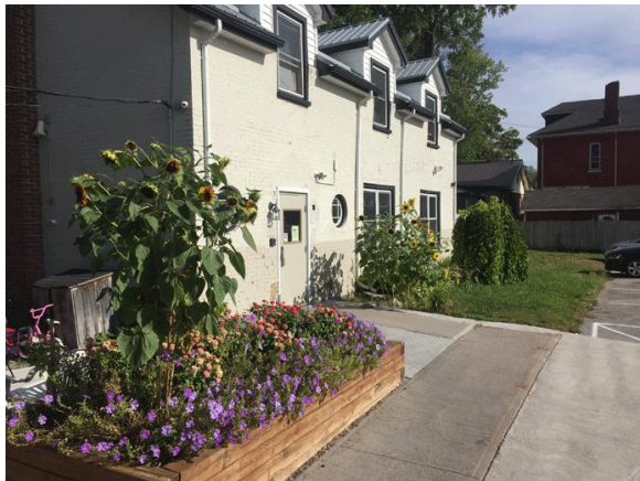
East Shelter Building
